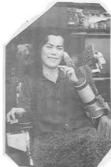
Figure 13. Successfully developed active arm orthosis for the rehabilitation of advanced cases of dystrophy and similar diseases. Controlled by means of a joystick. Made at the Mihailo Pupin Institute in 1982.
